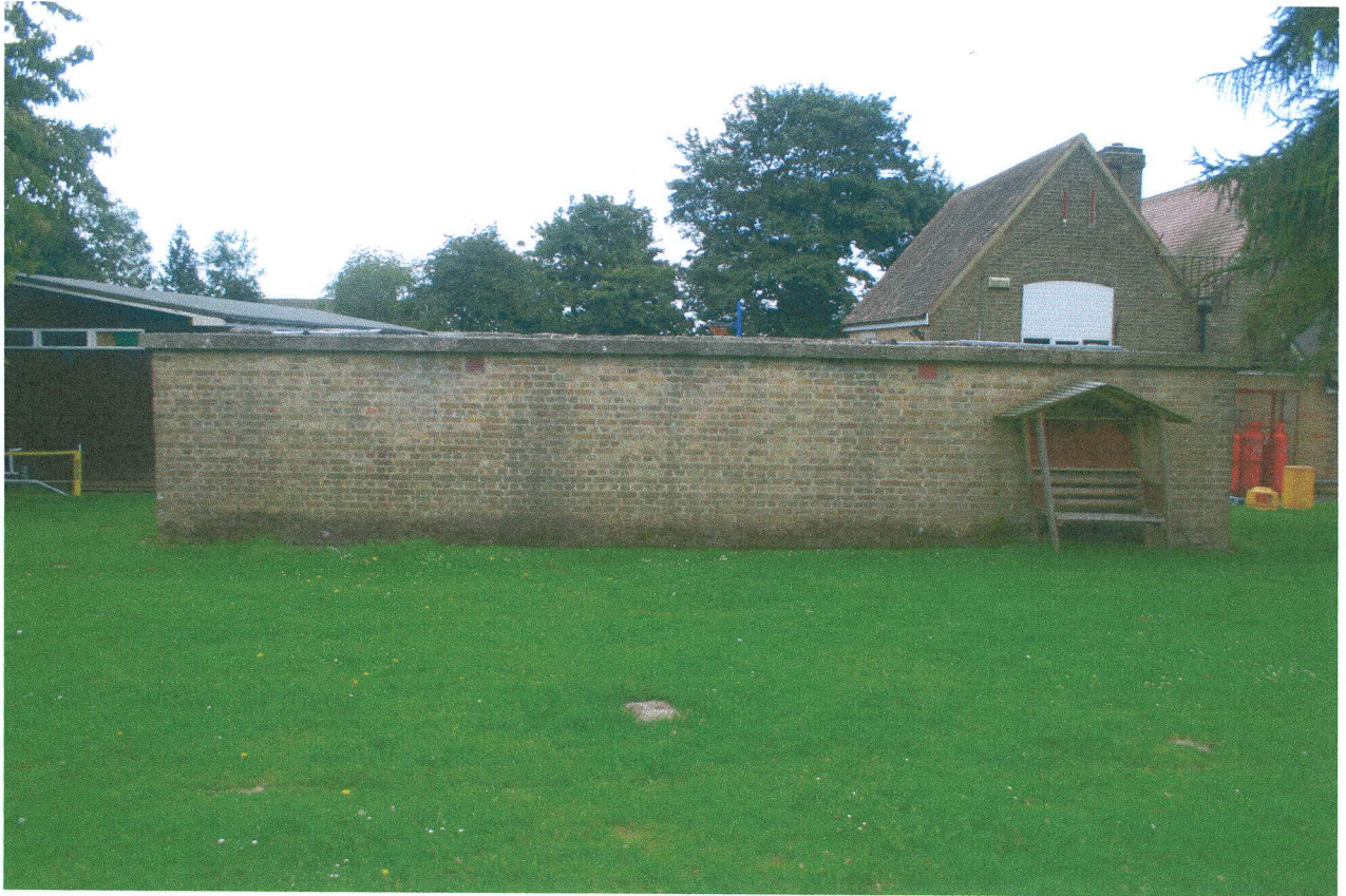
Air Raid Shelter. North West elevation.
