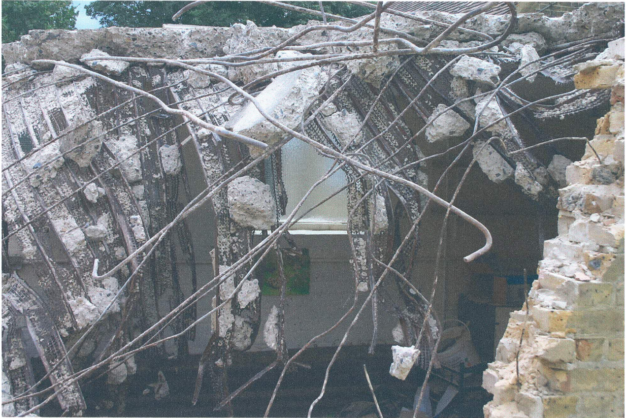
Air Raid Shelter. Showing reinforcing steel in roof.
