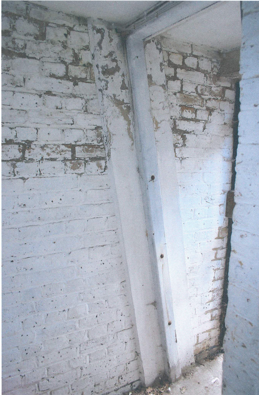
Air Raid Shelter. Internal view showing gas curtain frame.
