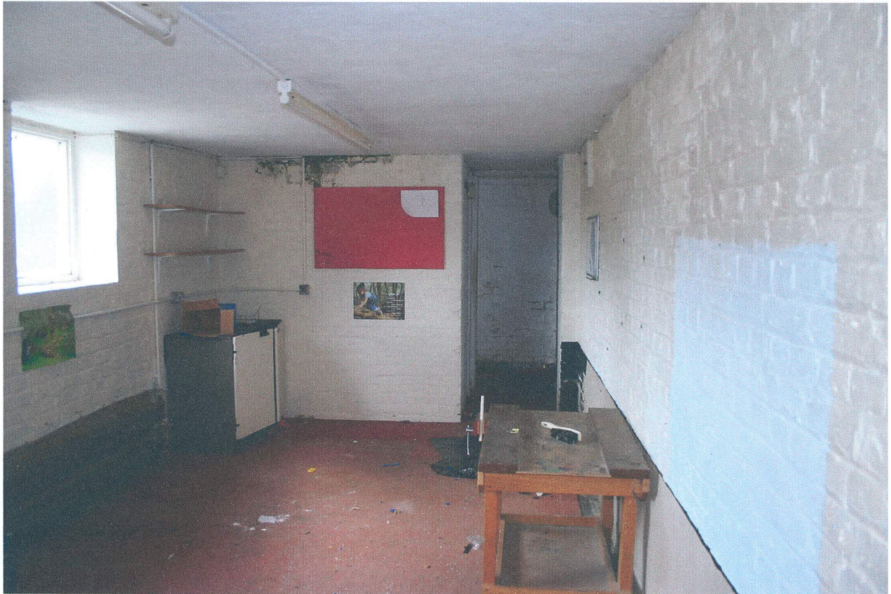
Air Raid Shelter. Internal view.
